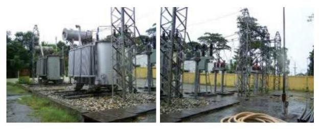
Figure 2-15: Open Transformers 33 kV / 11 kV / 415 V behind MPA Service Yard [Consultant]
