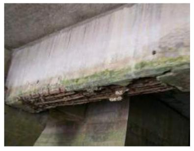
Figure 2-6: Damage of Beam [Consultant]
