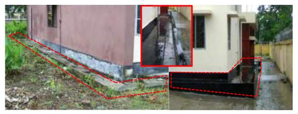
Figure 2-23: Typical Drainage Trenches around Houses [Consultant]
